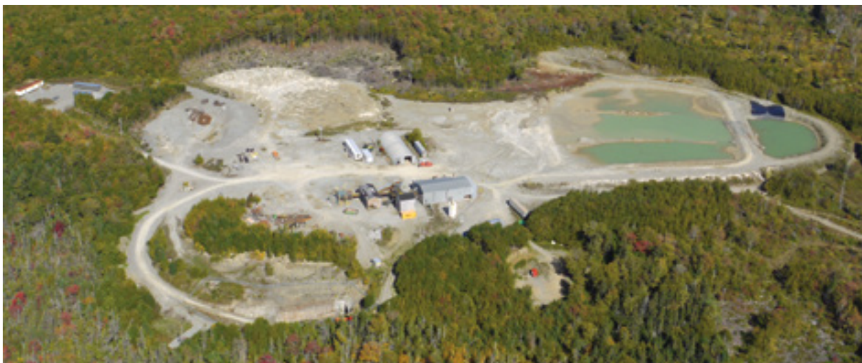
Figure 53. Aerial view of the Dufferin Mine site, near Sheet Harbour, N.S.
