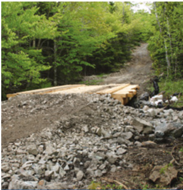
Figure 51. An exploration access road and bridge.
