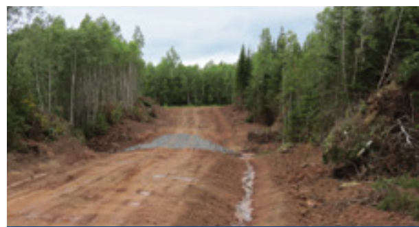
Figure 42. Proper road construction is essential in controlling erosion.
