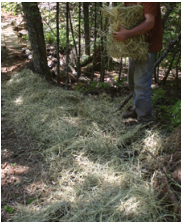
Figure 43. Erosion and dust can be reduced by placing straw in critical areas.
